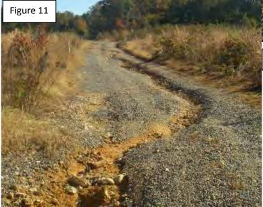
Figure 11: Lateral erosion across the roadbed, see #2.
