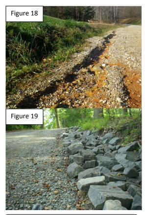
Figure 18: Accumulation of loose materials along the shoulder or in the ditch does not allow runoff to sheet off the roadbed.
