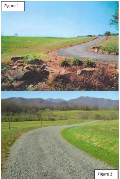
Figure 1: Gravel driveway directing runoff to stream crossing. Figure 2: Well-maintained gravel driveway
