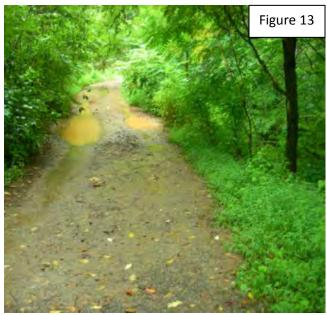
Figure 13: Massive ruts formed in a dirt road. The soils are soft and should be reinforced with Geotextile and need additional surface aggregate.
