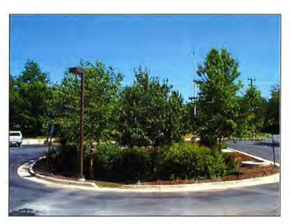
Figure 1: Bioretention created in a parking lot turn-around
