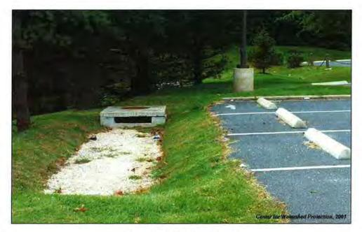
**Figure 1: Infiltration Trench**
