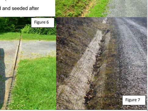
Figure 5: Elevated (In-slope) Gravel Driveway to inside ditch.Figure 6: Open top Culvert; Figure 7: Temporary stabilization matting in ditch
