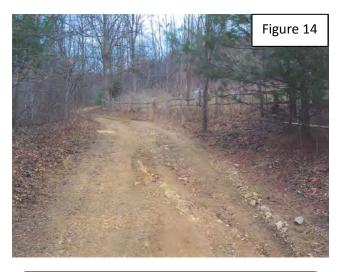
Figure 14: Runoff is conveyed down the driveway. The runoff needs to be diverted to a side ditch. A Dip or Diversion can be used; see the practice specifications.
