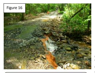
Figure 16: Frequent high flows that can clog and overtop the roadbed need a high water bypass; see practice specifications.
