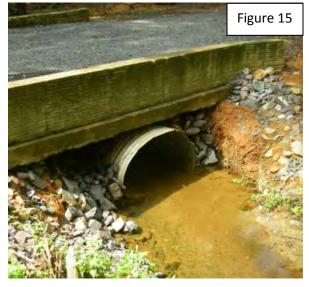
Figure 15: Inadequate culvert bedding combined with high flow depths causes piping; which is the loss of fill material. A headwall or riprap lining is needed.
