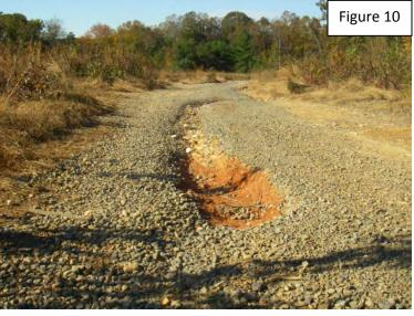
Figure 10: Erosion down the roadbed, see #1.
